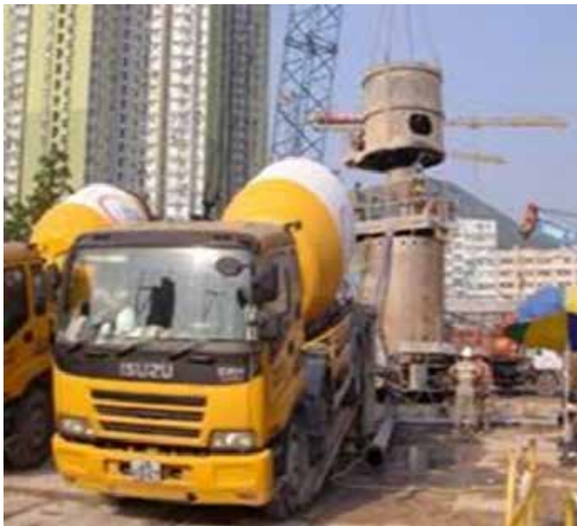
Figure 5. 21 Concreting Bored Pile
