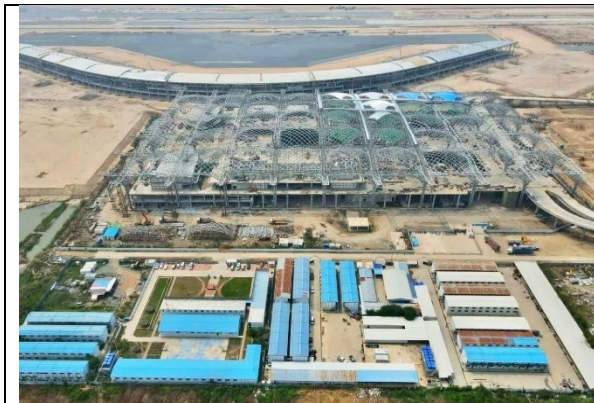
Image: Techo Takhmao International Airport Source: Heerim
