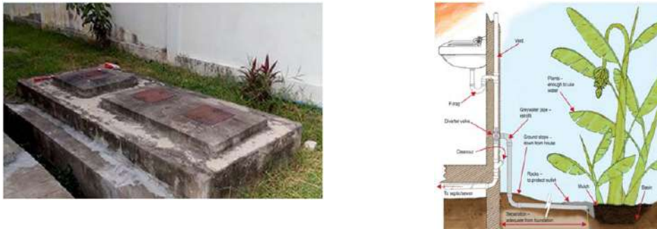
Figure 4.3-13 Septic Tank and Gray Water Disposal Plan
