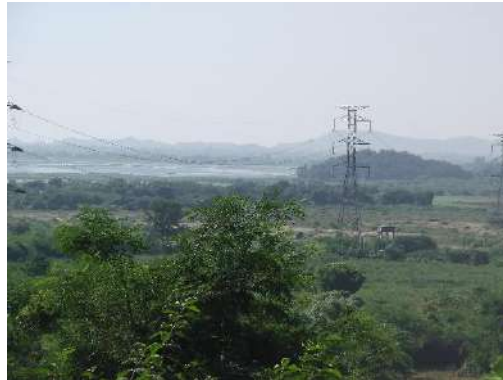
PHOTO 5.4.2-12 : EXISTING LAND USE ALONG THE PROPOSED TRANSMISSION LINE ALIGNMENT
