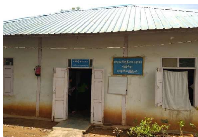
PHOTO 5.4.5-5 : KYAUNG SUB-RURAL HEALTH CENTER, KYAUKSE TOWNSHIP
