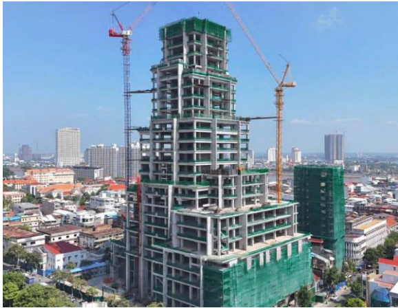
Picture: The National Bank of Cambodia's Headquarters under construction Source: Ultracon
