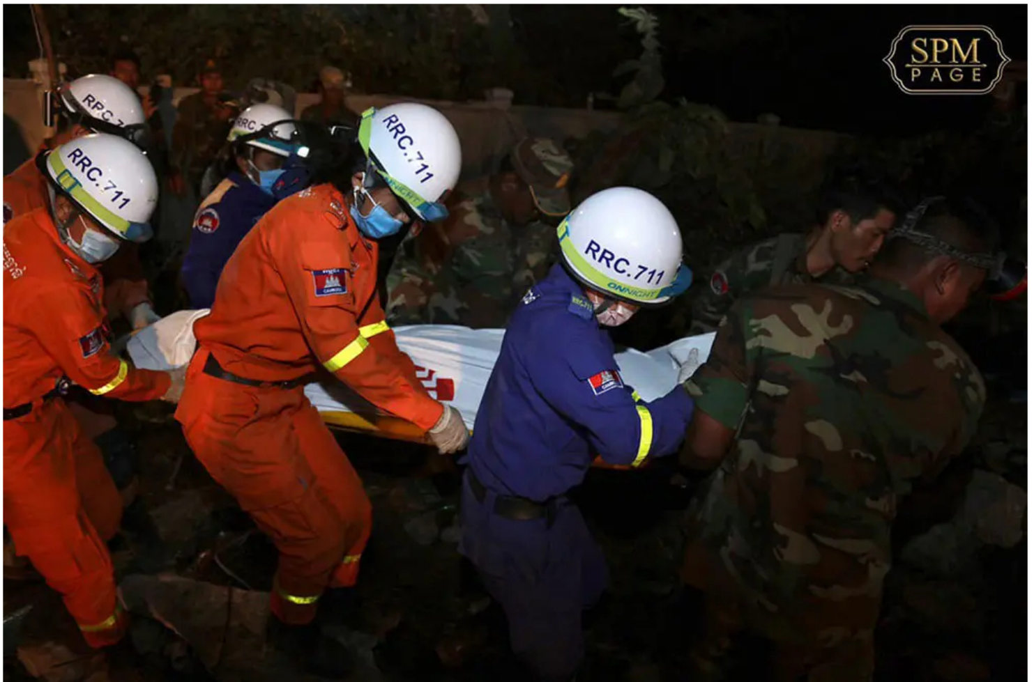
The rescue team carry a dead body from collapsed building in Kep province. Supplied
