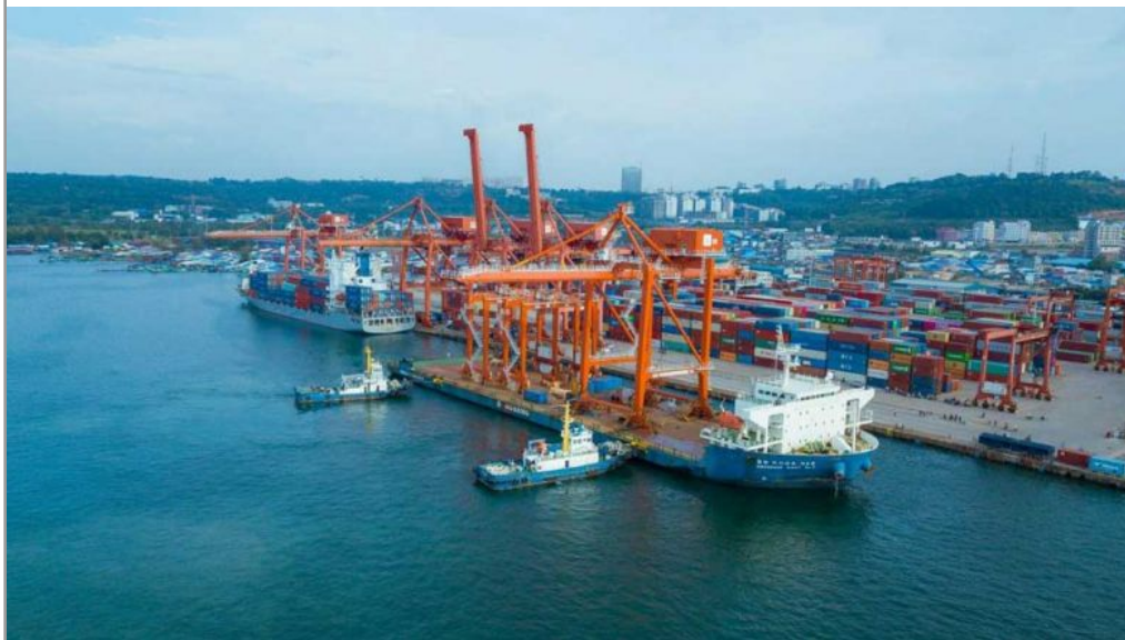
The Sihanoukville Port Urgent Rehabilitation Project was launched in 2002. Photo supplied
