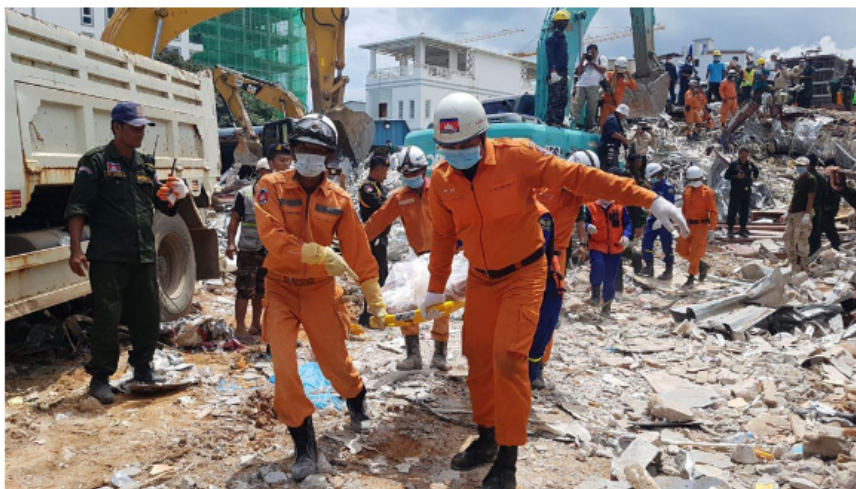
The building collapse in Sihanoukville killed 28 people and injured 26 on June 22 last year. facebook
