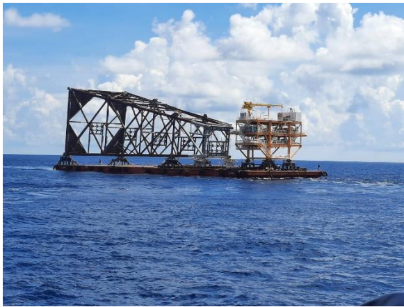
Load out of the topsides of the Apsara Mini-Platform
