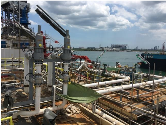
Process pipework on deck of Ingenium II production barge
