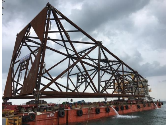
Load out of the jacket structure of the Apsara Mini-Platform
