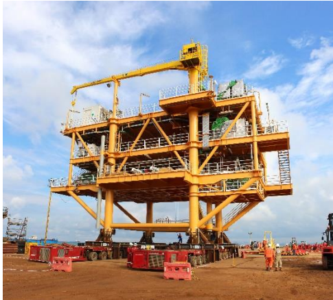
Load out of the topsides of the Apsara Mini-Platform
