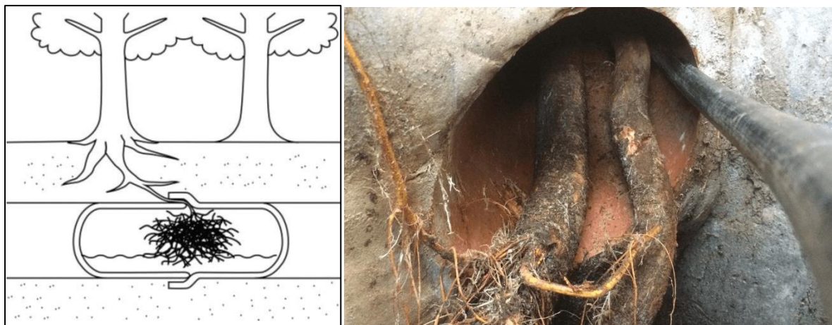
Figure 4. Tree roots in sewers
