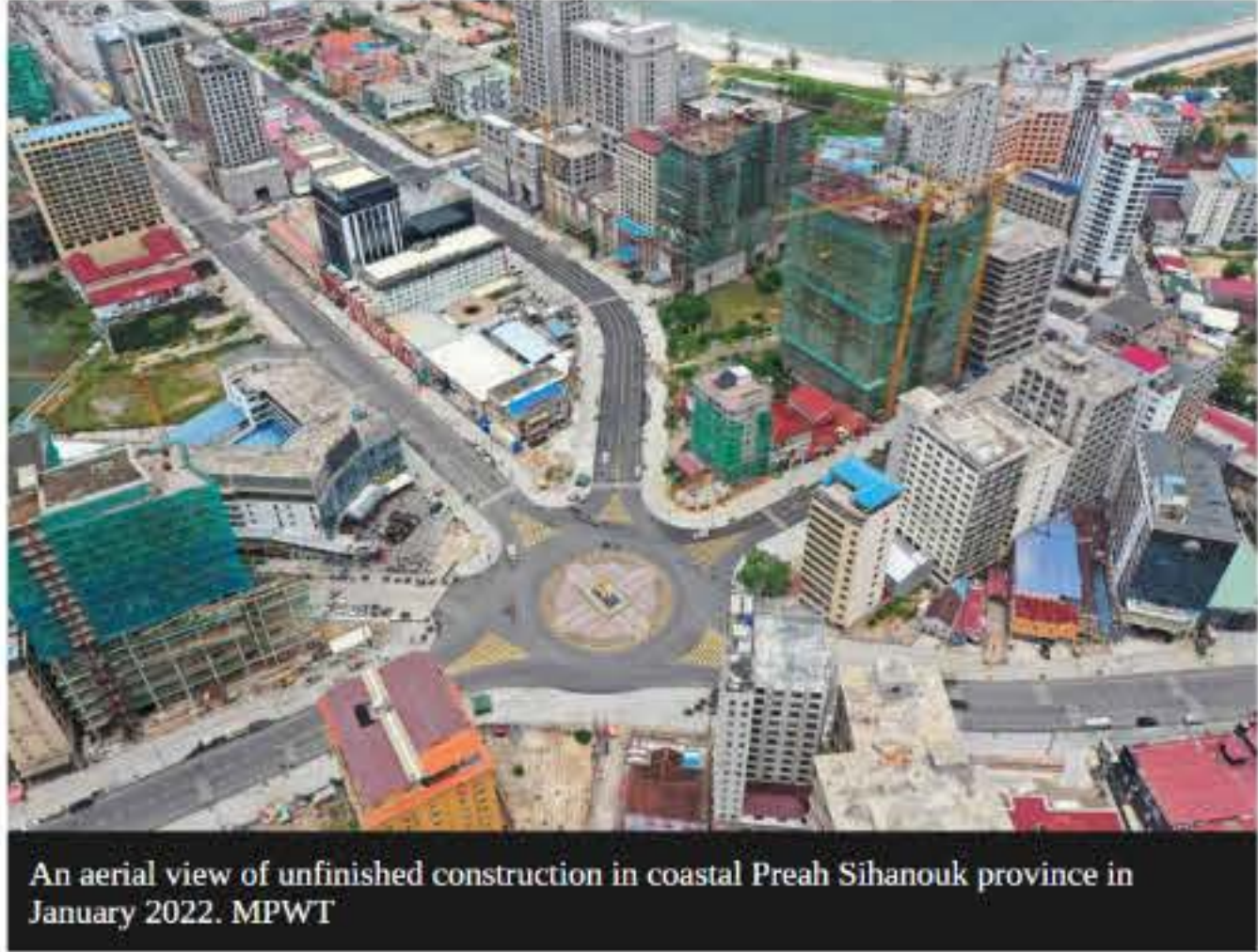
An aerial view of unfinished construction in coastal Preah Sihanouk province in January 2022. MPWT
