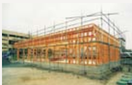
Store under construction
