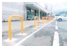
Parking Lot Guardrails
