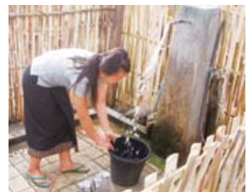
Water supply facilities in Laos
