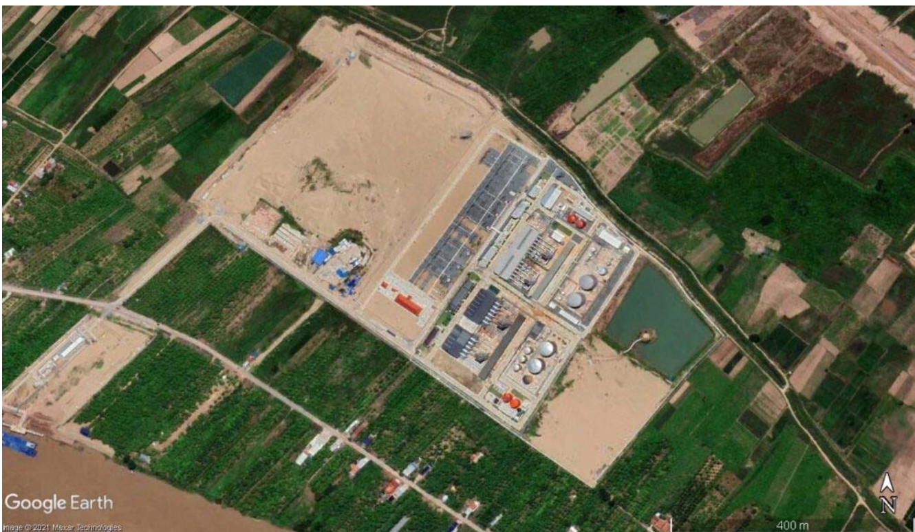
Satellite image of power plant, June 2021. Source: Google Earth.
