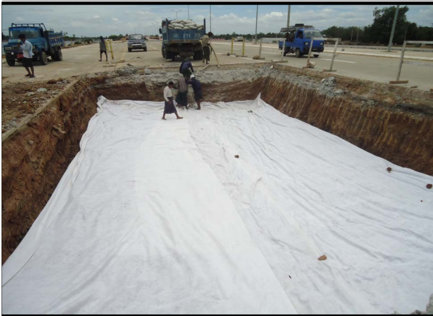
Reconstructing the Expressway by paving the Geotextile layer near mile post 366
