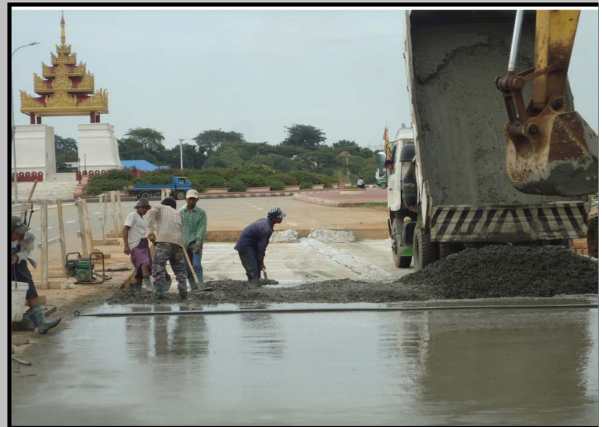
Reconstructing the Expressway by paving the Geotextile layer near mile post 366
